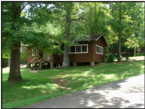
Cabin at Piney Creek Camp
