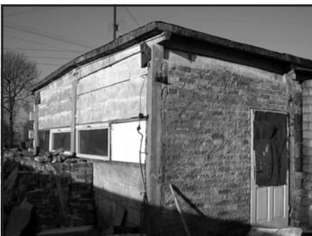
The outside of the garage turned print shop
