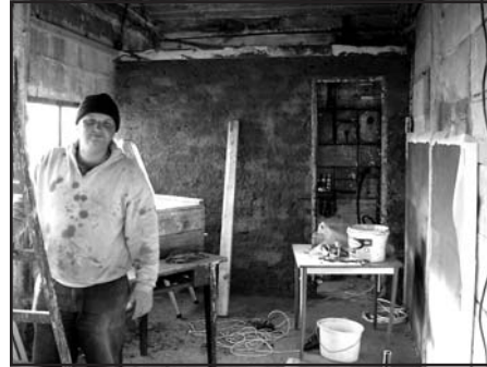
Rafal beginning the remodeling work on the garage
